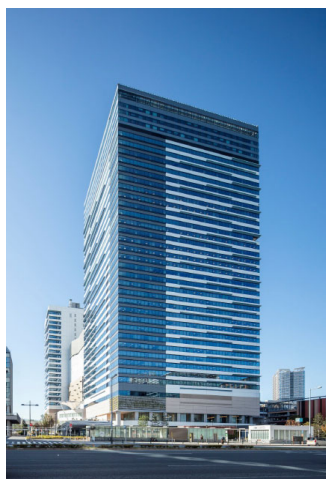
Source: "Nippon Building Fund Inc." HP
