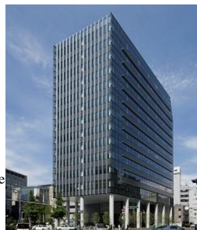
Source: "Nippon Building Fund. Inc." HP
