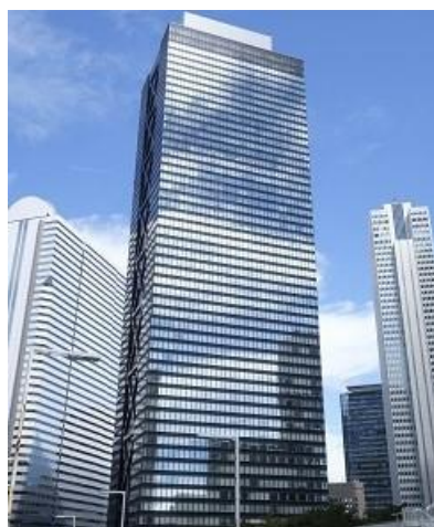
Source: "Nippon Building Fund. Inc." HP
